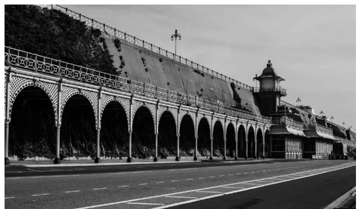
The Victorian iron work before the elements took their toll
